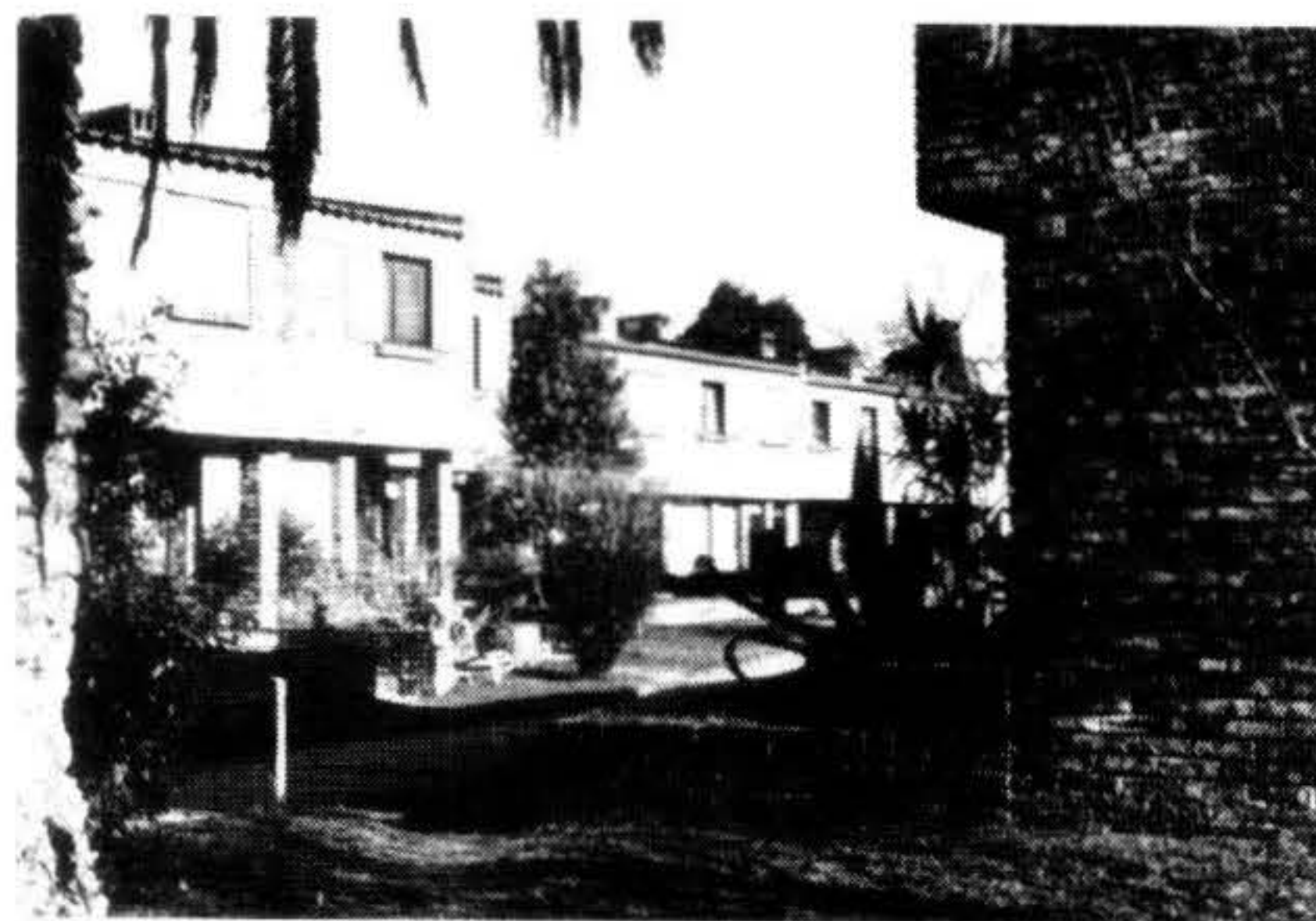
Covimt 1 (calle Schiller, Peñarol)
