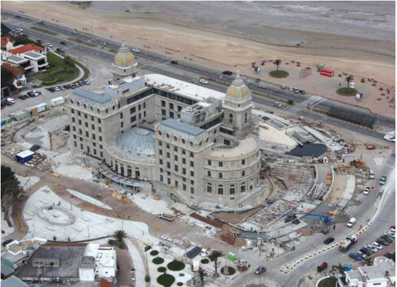
Remodelación del Hotel Casino Carrasco, en obra. Renovation of the Hotel Casino Carrasco, construction work in progress. Montevideo.
